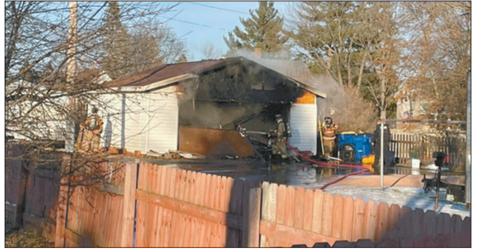
The scene of a Sunday afternoon garage fire in Merrill's Sixth Ward. Photo courtesy of Merrill Fire Department.
