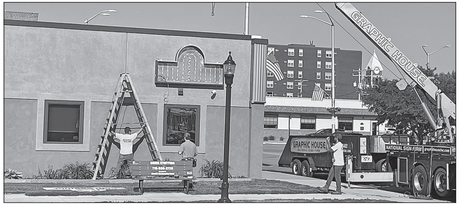
New signage being installed at Merrill Community Bank, now known [along with Tomahawk Community Bank] as Crossbridge Community Bank. Tina L. Scott photo.
