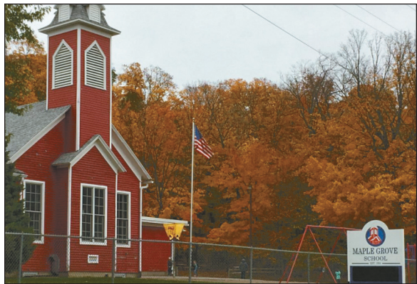
Maple Grove School, including the building and acreage, has now completely transferred to the School District of Athens. Submitted photo.
