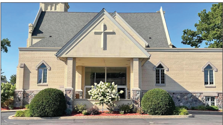
Trinity Lutheran Church is located on the corner of West Main and State Streets in Merrill. Tina L. Scott photo.
