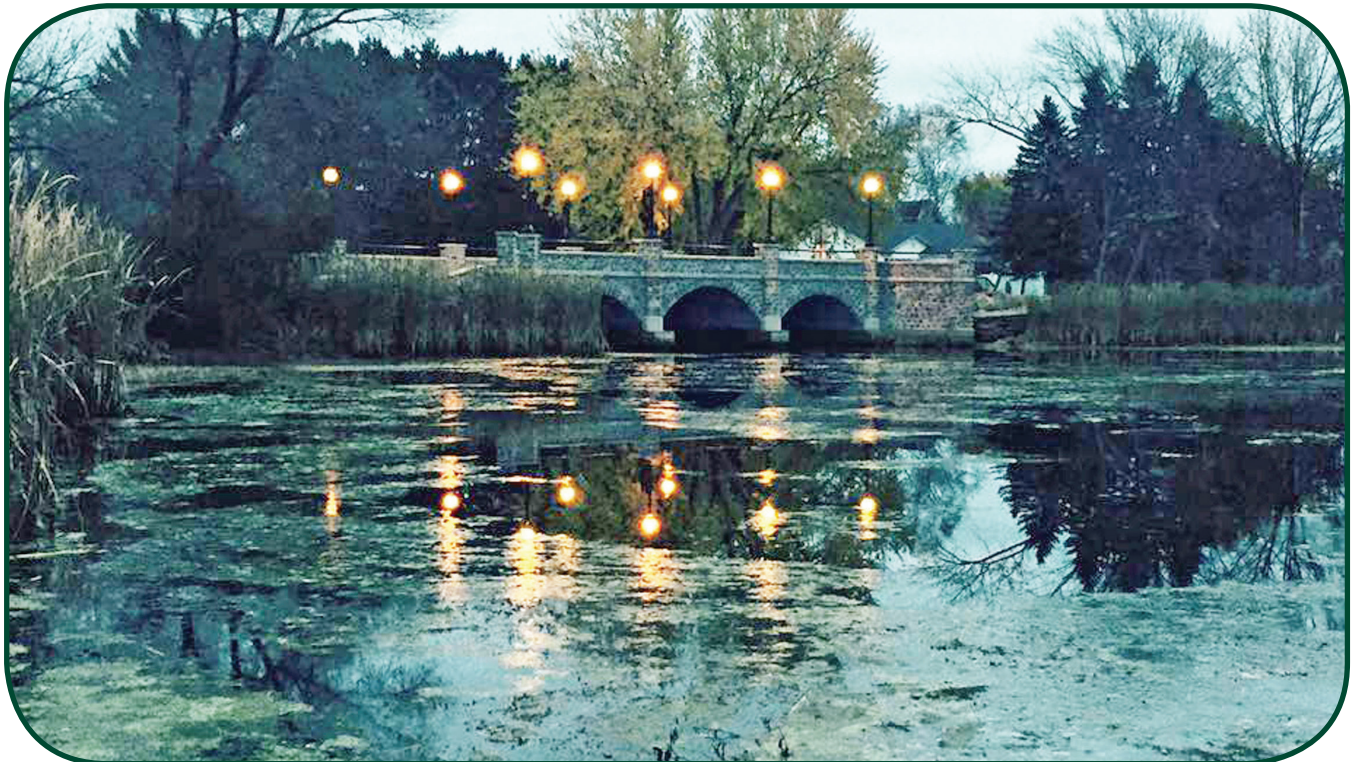
Hudson Street Bridge, Antigo
