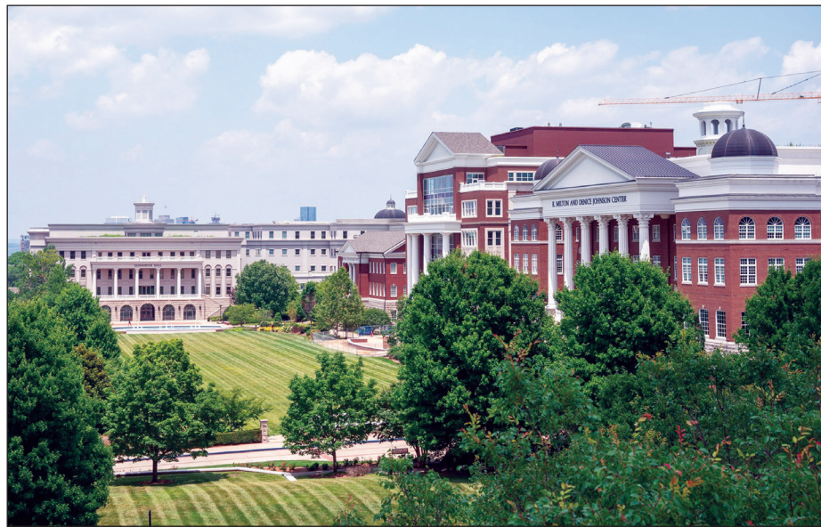
The main campus buildings of Belmont University in Nashville, Tennessee, June 27, 2023. Photo by Sam Simpkins
