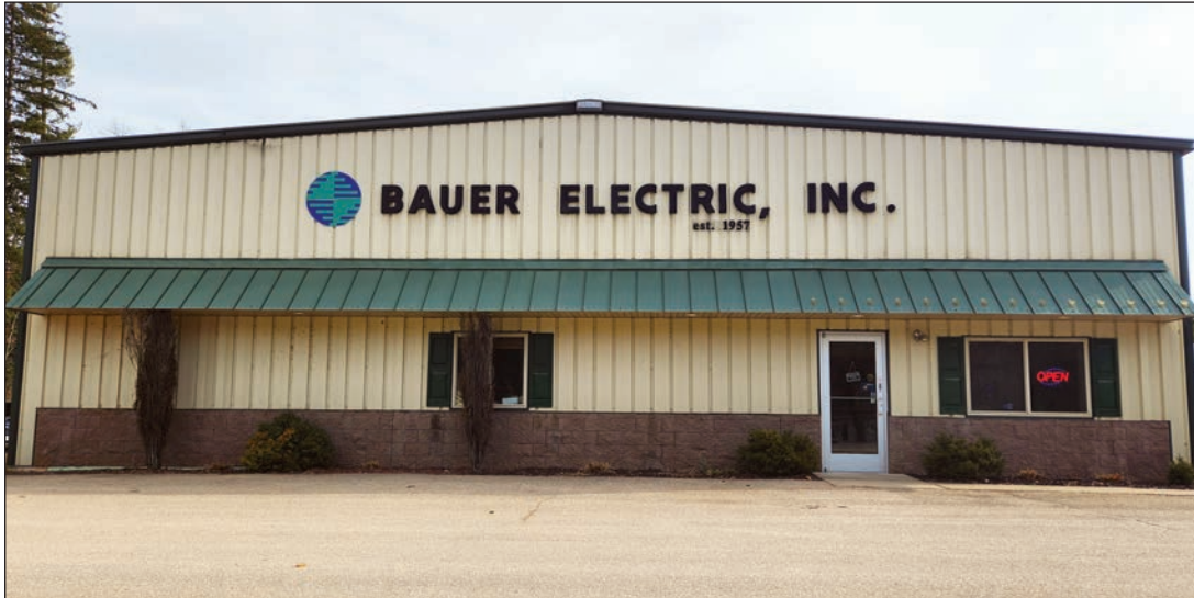
Bauer Electric is located at N2858 County Trunk QQ in Waupaca.
