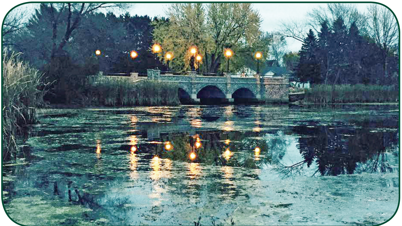
Hudson Street Bridge, Antigo
