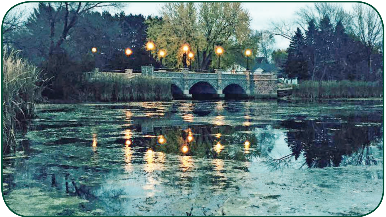
Hudson Street Bridge, Antigo
